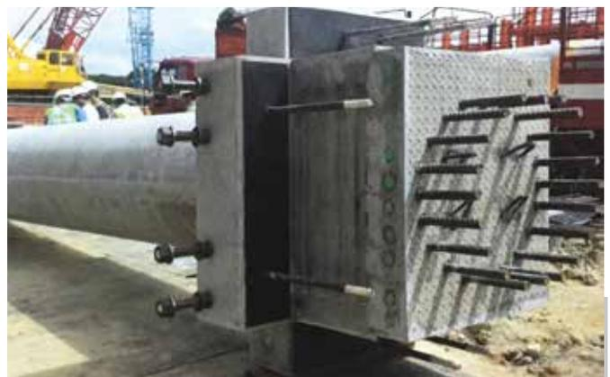
A full precast system with mechanical beam shoe connectors was adopted in the project - the first of its kind in Singapore. The system was chosen in view of its buildability and flexibility for future upgrading of the airport.
