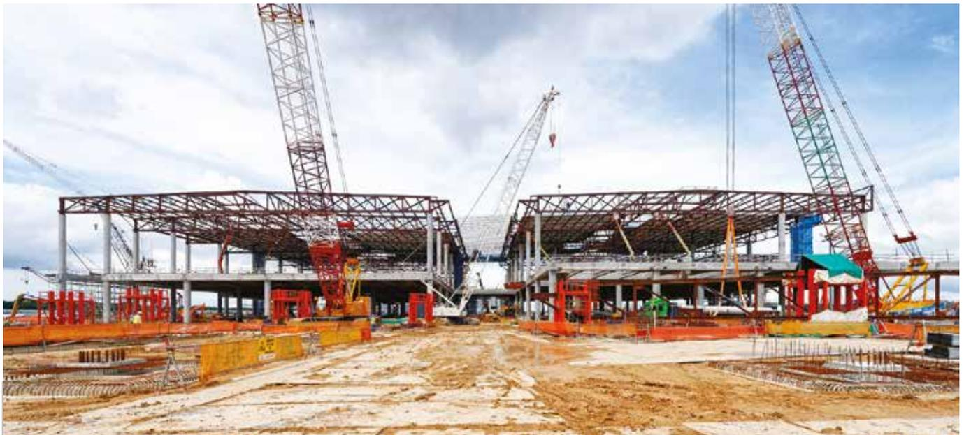
The sloping top-chord pitched trusses supporting the terminal roof were also prefabricated offsite.
