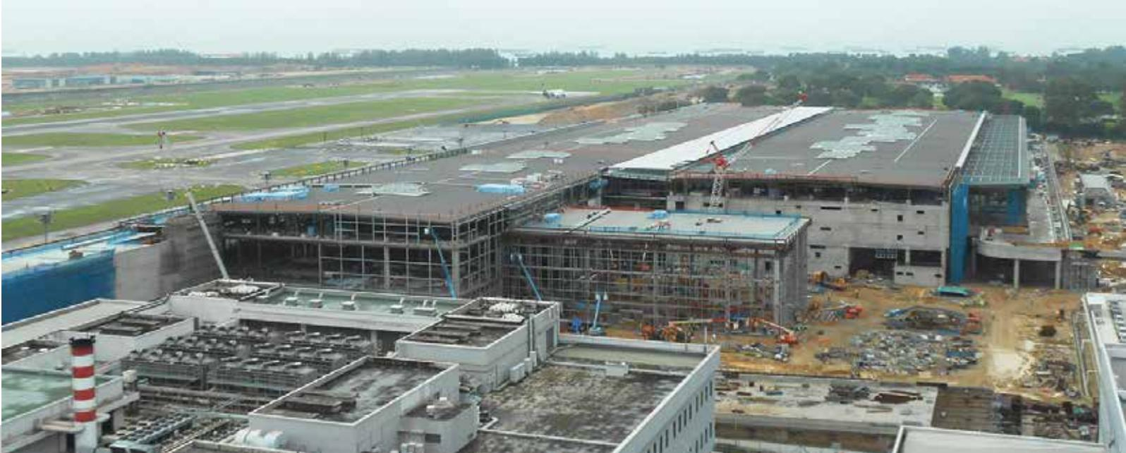
The project team implemented the 'hat-first' construction method for the main terminal building. The second storey and roof were completed first, then works continued on to the first storey and Mezzanine floors - starting at the centre of the building and moving outwards. This approach allowed the internal finishing and M&E works to start quickly, and also enabled an early installation of the baggage handling system.
