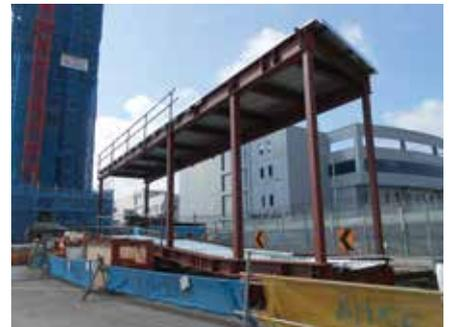
Fixed gangways were prefabricated offsite and assembled onsite – two at a time and without any welding works. This method improved productivity in general.
