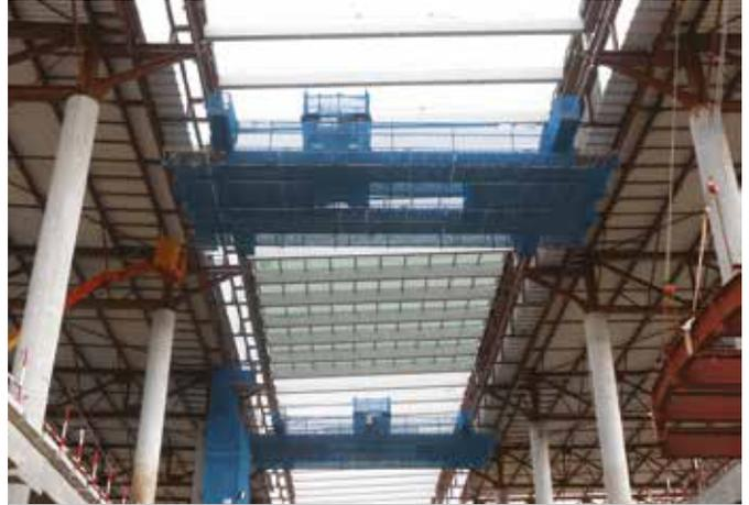
'Magic carpets' being used to install glass panels on the Galleria Skylight. These mobile hanging platforms were able to move along the entire roof safely.
