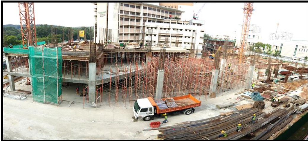
Construction Progress for Thomson Hospital Kota Damansara Expansion – May 2019
