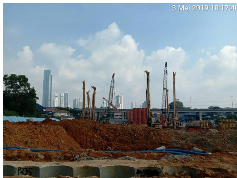
Piling works progress for Thomson Iskandar Medical Hub – May 2019
